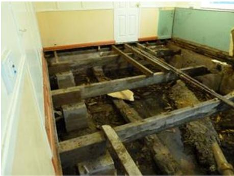
The horror of discovering an unexpected lake, an assumed drainage pipe, and the sight of the flooring joists so badly rotted that they were not all on the pier supports. The floor was **near total collapse** - in fact it was lucky it had not collapsed over the recent months as slope and bounce had got greater.
